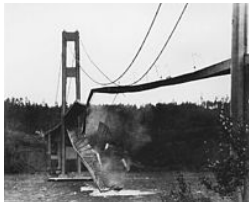
Tacoma Narrows Bridge Collapse November 7, 1940
