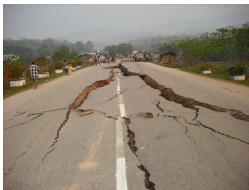
Cracked road after Burma's earthquake March 24, 2011
